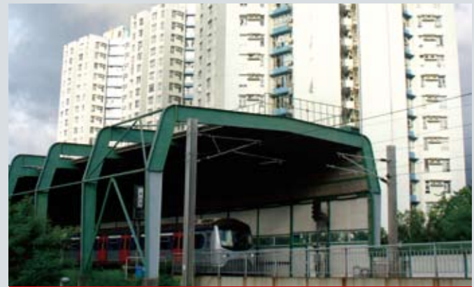
Semi-enclosure to protect residents from train noise.
